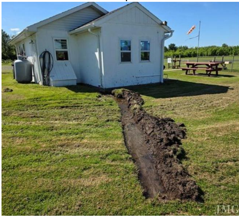
Trench work at the corner of the pavilion on 08 June:
